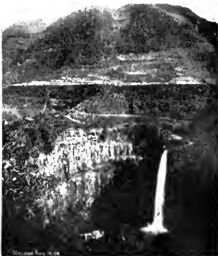
First Necaxa Falls, showing temporary plant.
